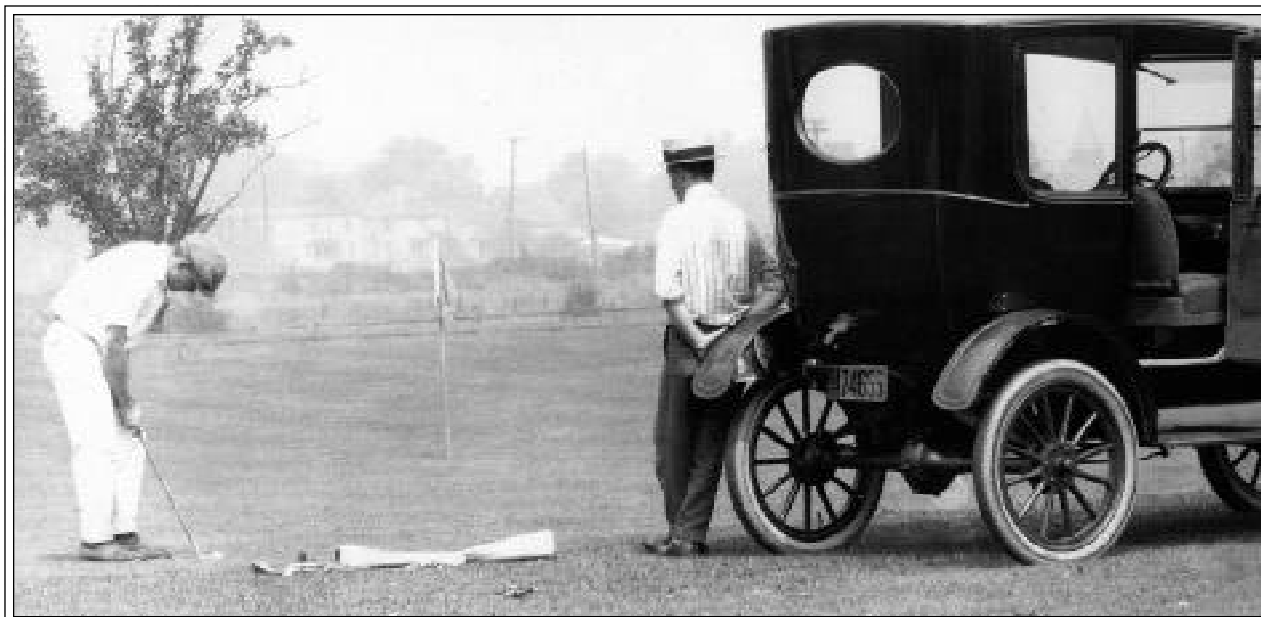
This photo of golfers on the Prince Farm course was taken for an advertisement for Ford Motor Company of Canada in 1919. Note the church steeple through the car window.
